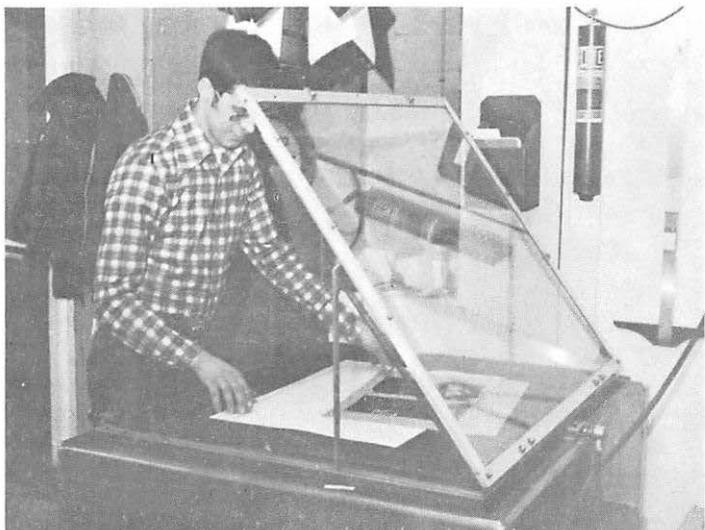
Bob Sallee “burning” image from negative to metal press plate
